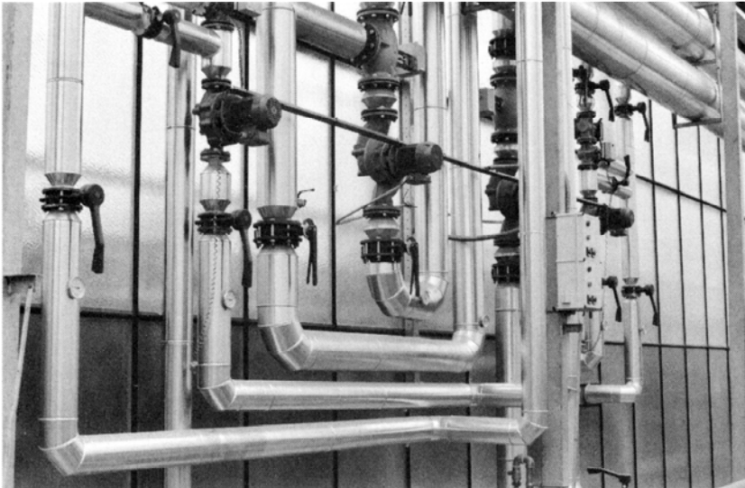
Large CO2 dispersing unit in commercial setup. Photo ©Crop King
