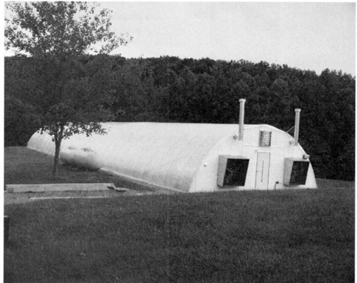
Fans help exchange and cool the air in this unit. Photo ©Crop King
