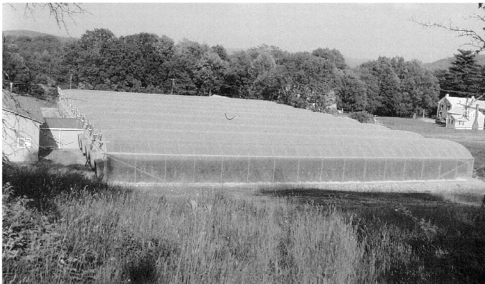
Small family run setup, cooled and heated.
