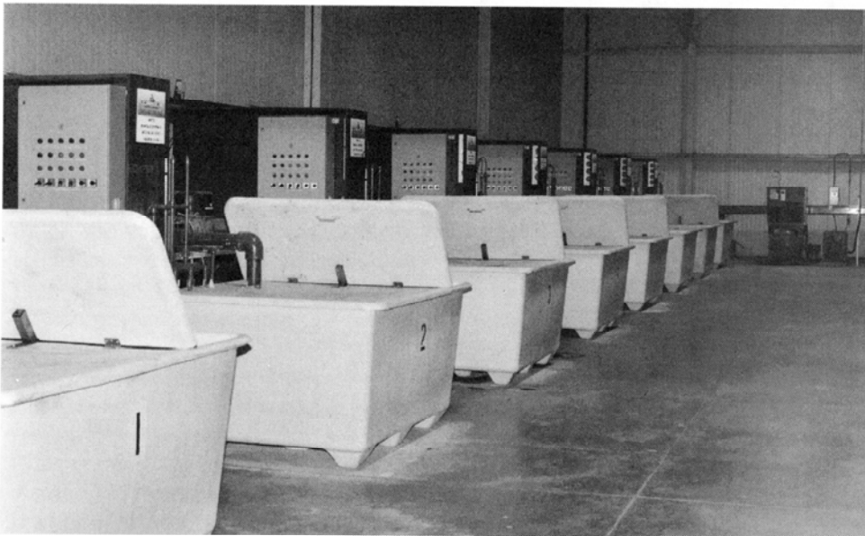
Commercial nutrient mixing and delivery systems.
