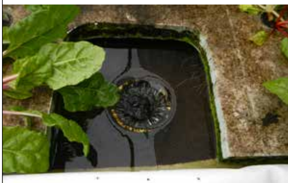
FIGURE 9.14 Stand pipe in a deep water culture canal maintaining the water column height
