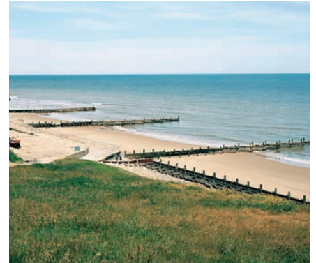
▲ Figure 15 These shoreline groins prevent beach erosion by trapping sediment.
