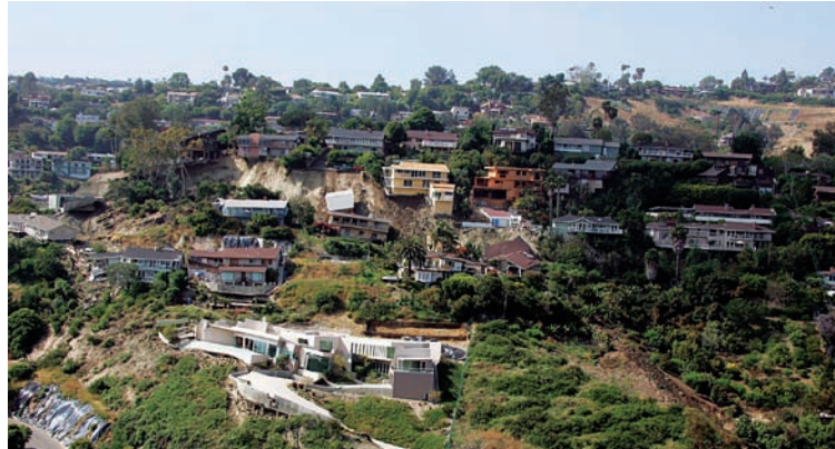
Figure 20 Building on steep slopes can increase the risk of a landslide. Construction or removal of vegetation makes the hillside even less stable.
