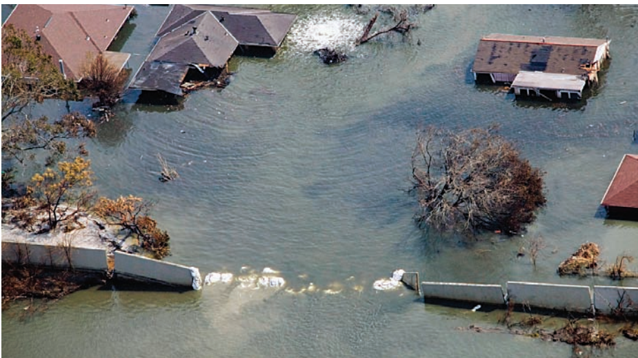
◀ Figure 16 This 2005 levee break in New Orleans caused extensive flood damage.
