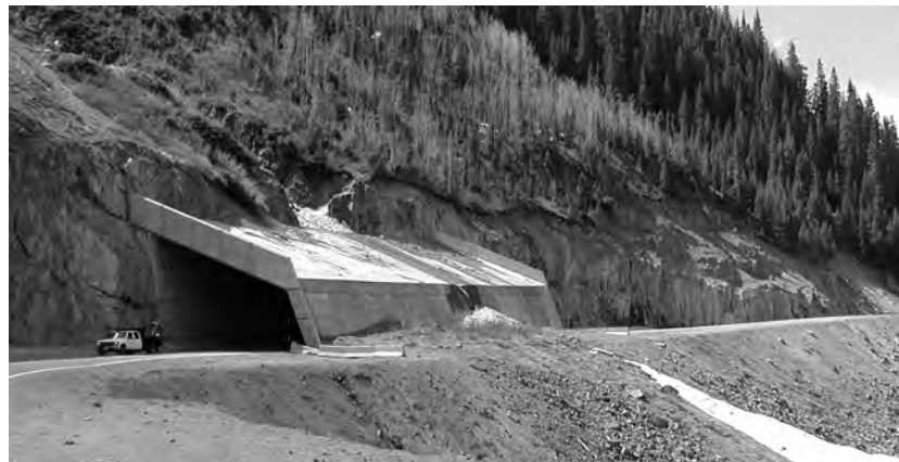
Figure 9-8 This snow shed in the Rocky Mountains protects the road and people who travel on it from avalanches and landslides.
