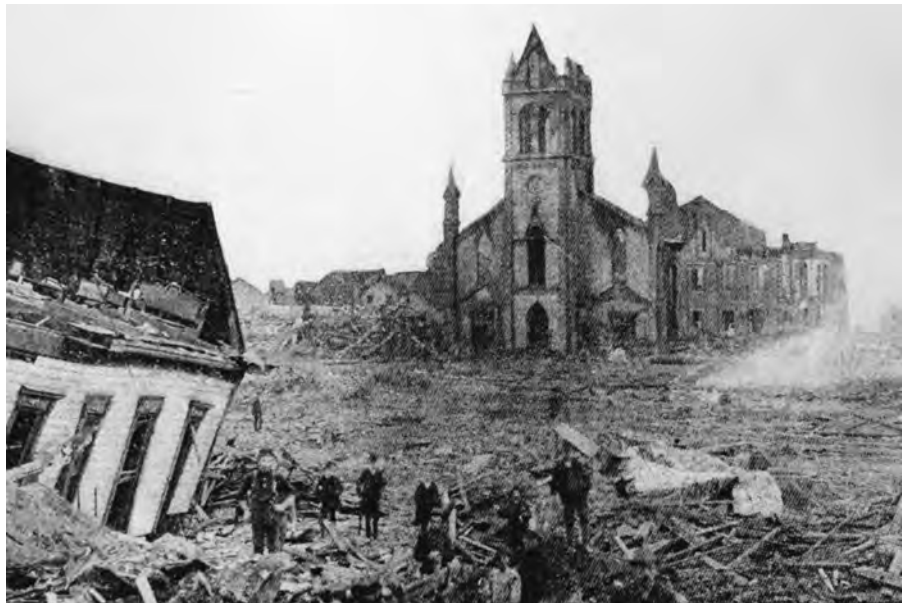
Figure 23-1 Damage caused by the 1900 Galveston Hurricane.
