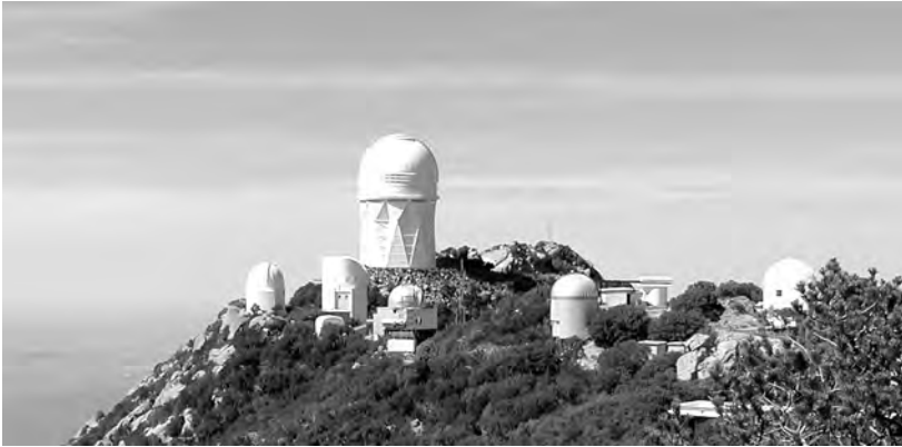
Figure 28-4 The telescopes of the Kitt Peak Observatory are located on a mountaintop to reduce problems associated with light passing through the atmosphere. The higher the observatory and the farther it is from atmospheric pollution and artificial lights, the better the quality of the observations and images.
