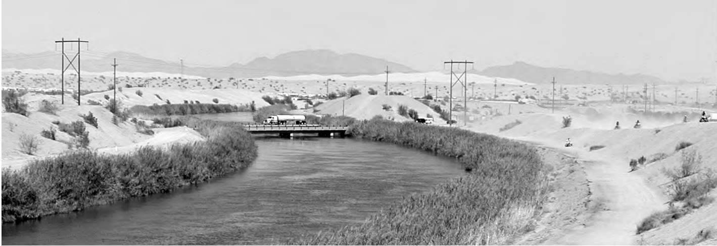
Figure 6-5 This canal diverts a major part of the Colorado River into the Imperial Valley of California. Normally, none of the river's water reaches the Pacific Ocean.
